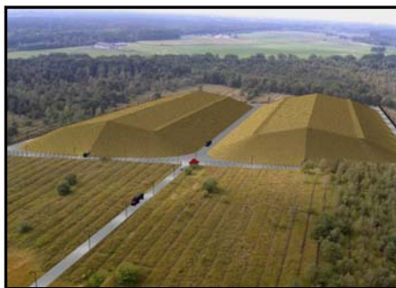
Figure 1.2-7 Sealed modular trench repository with built multi-barrier protective cover; (a) exterior; (b) protective cover details
