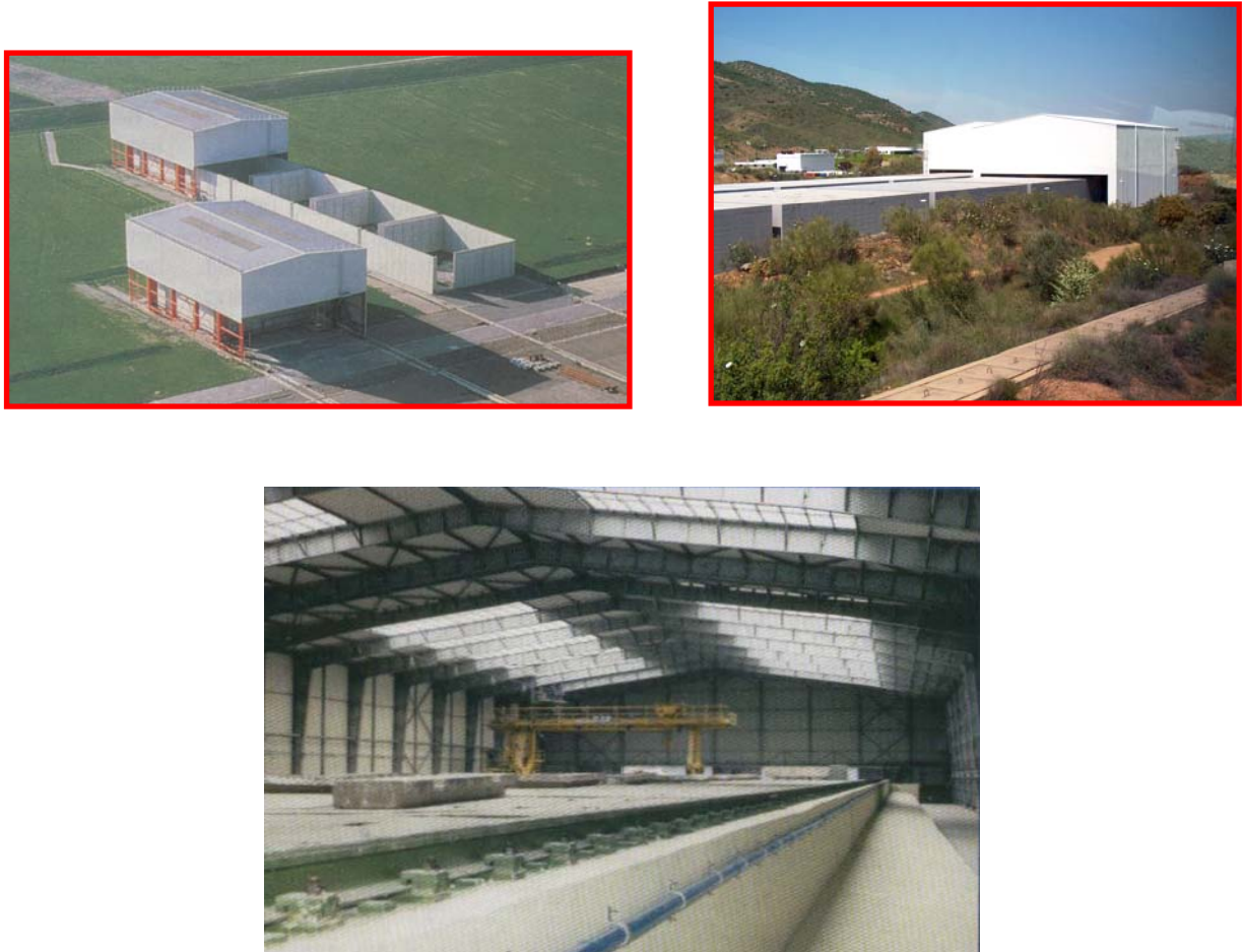
Figure 1.2-9 Modern repositories for low and intermediate level RAW with protective constructions during the operational period: (B) Mochovce, Slovakia
